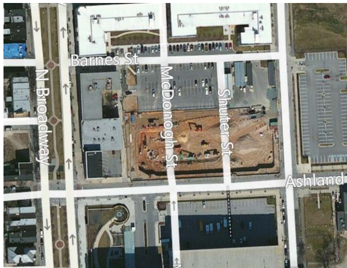
Figure 4: Site Aerial View (image provided by Bing.com)
