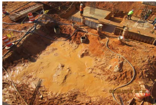
Figure 28: Flooding in Excavated Site (image provide by Jacobs Engineering)
