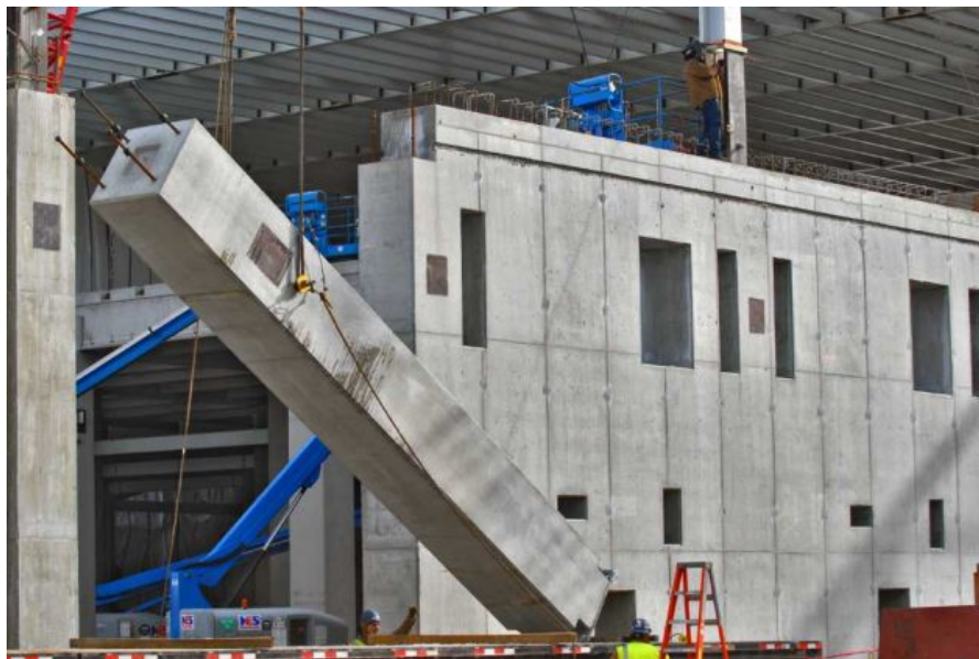
Figure 5: Precast Column Erection (image provided by timesunion.com)
