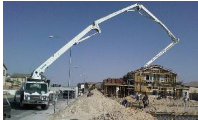
Figure 10: Grout Delivery Truck and Pump (image provided by all-concrete-cement.com)
