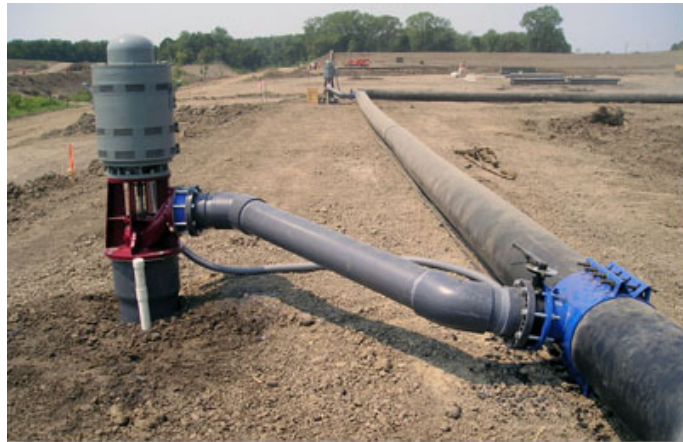
Figure 29: Deep Well Dewatering System (image provided by Griffin Dewatering Co.)
