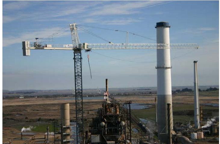
Figure 8: Hammerhead Tower Crane (image provided by Biggie Crane and Rigging)
